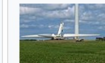
Wind turbine blade assembly being prepared for installation near St. Leon, Manitoba.
